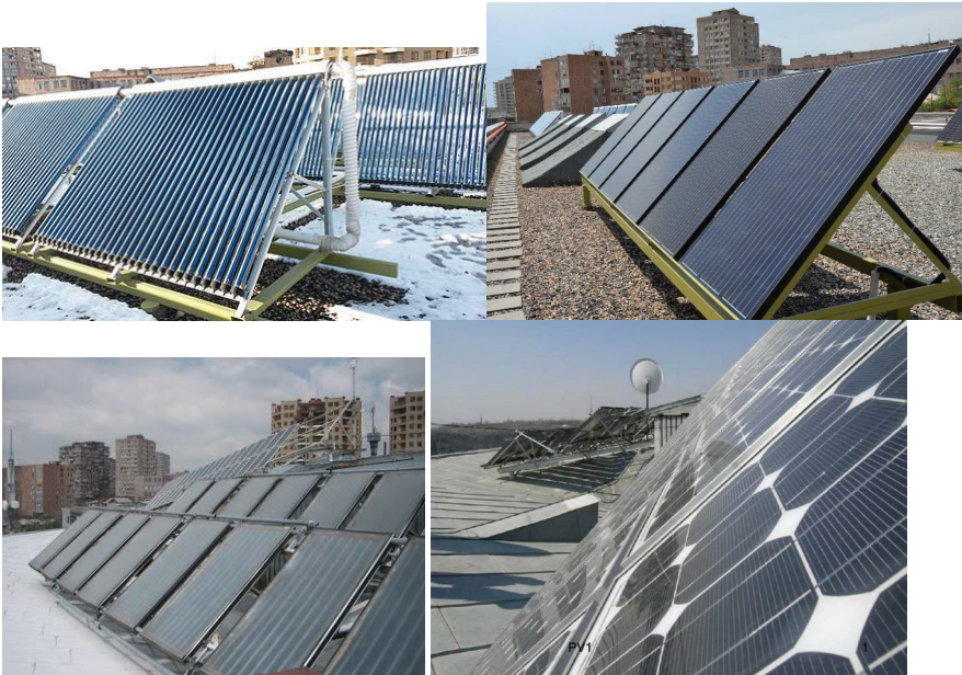
Figure 3.5. Comparison of PV and SWH panels installed on a support structure. Please note that on the top right vacuum tube panels are shown.
