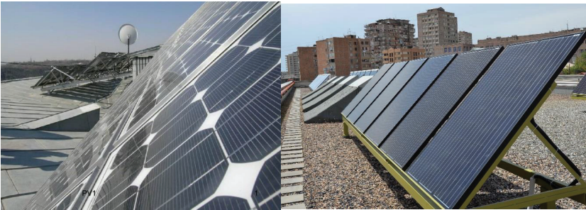
Figure 3.3. Solar PV modules. Note that solar cells cover not all the surface of the panels in the left picture, while the right panel has a higher “optical fill factor”. A support structure is needed for these rigid panels.
