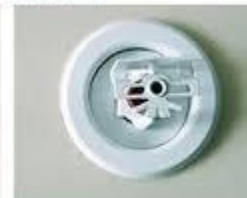
sidewall sprinkler
