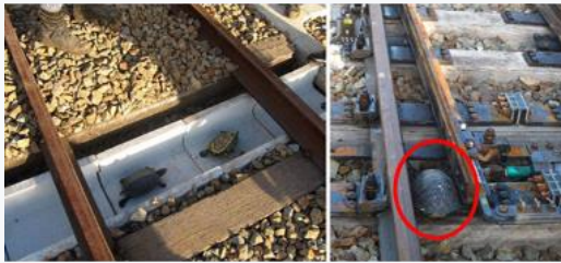
A turtle culvert under train tracks in Japan
